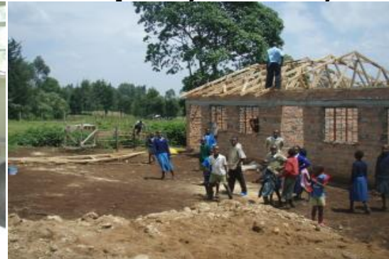
Classroom roof begins to take shape!
